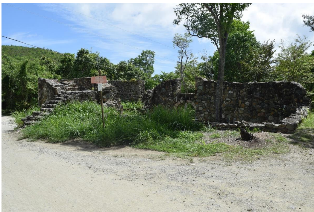
The factory, looking southwest (Source: Quinn Evans)
